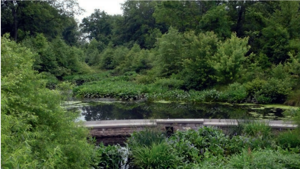
Case Study 8.2 Figure 1 Extended detention weir, Conference House Park, Staten Island Bluebelt.
