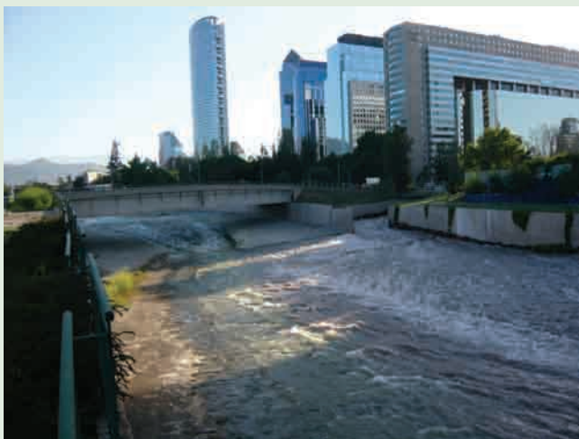
Box Figure 5.6: San Carlos channel (early nineteenth century) entry into the Mapocho River, an artificial channel that draws water from the Maipo River and takes it north into the Mapocho.
